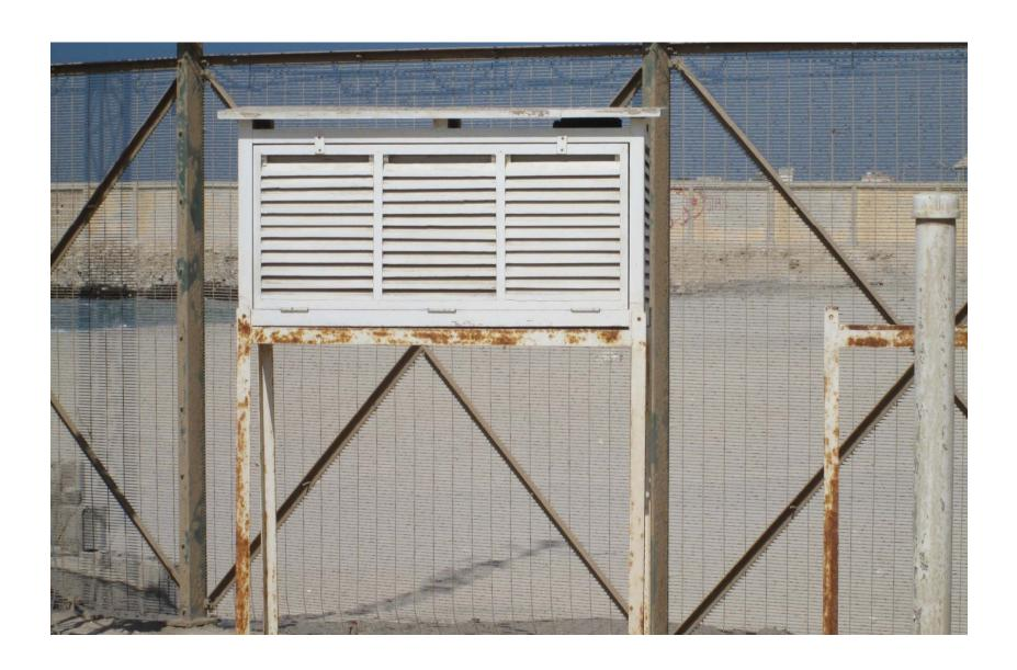
Another example of stations is  $\underline{TRINA}$ . That located in middle desert in south of Qatar. It has dust storm all the year and temperature reach around 50  $^{\circ}$  in the summer, so the more maintenance is needed. With sand and high Temp, the measurement process cant be in normal case with out of highly maintained.
